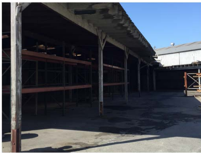
Structure B, C, H Open Storage Shed
