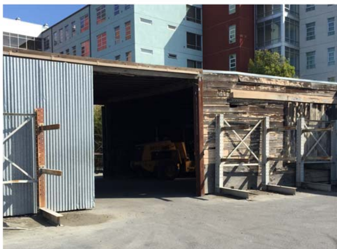
Structure D (rear) Open Storage
