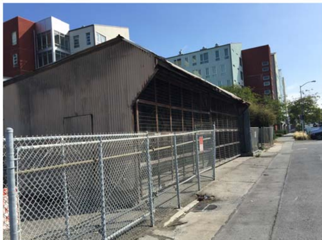
Structure F Open Storage Shed
