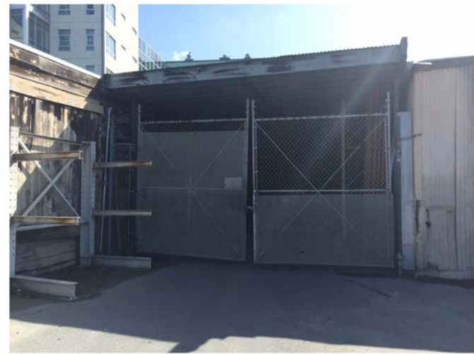
Structure D Open Storage Shed
