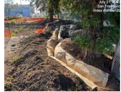
Root Protection for Trenches
