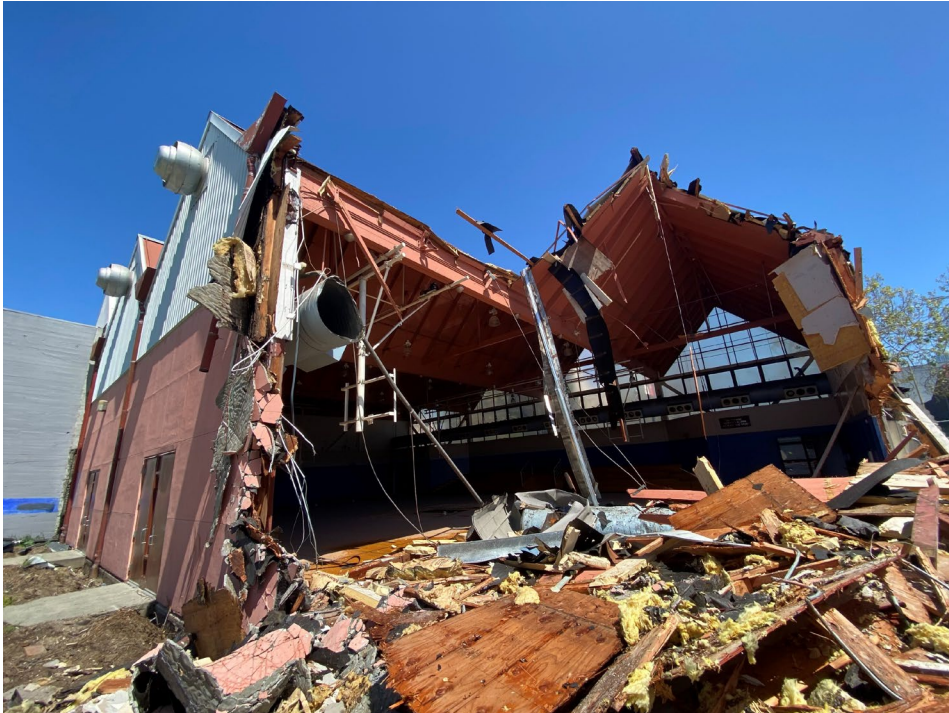
Demolition of the old rec center, in progress (Spring 2024)
