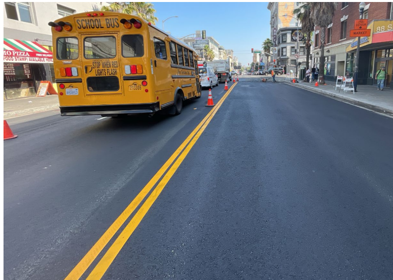
New Paving at 6 th and Mission
