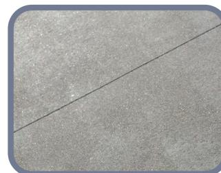
Cast-in-place concrete paving with silicon carbide and saw-cut joints
