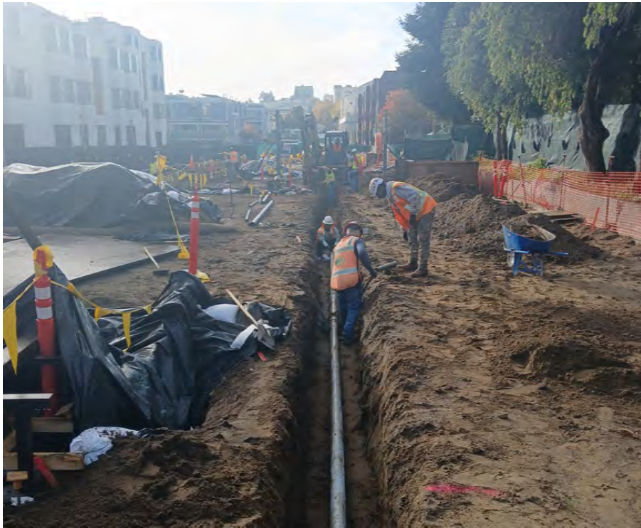
Irrigation mainline installation
