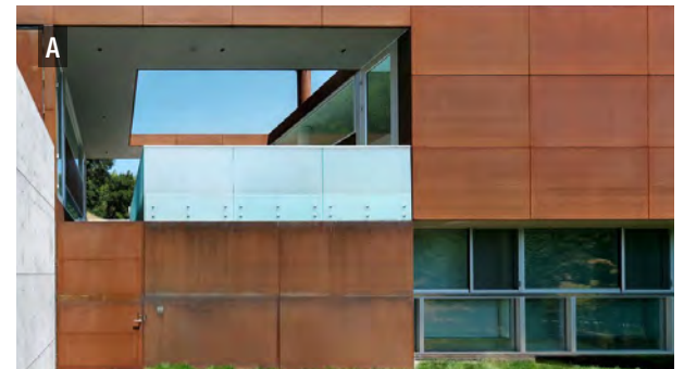
Corten steel or natural weathering steel
