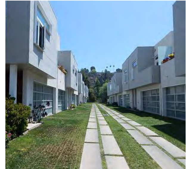
Permeable and vehicular rated paving is used to maximize pervious surface for stormwater management
