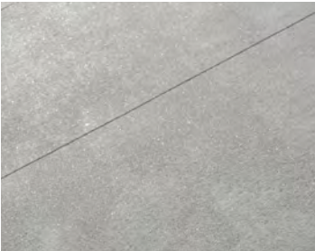
P1: cast-in-place concrete paving with silicon carbide and saw-cut joints
