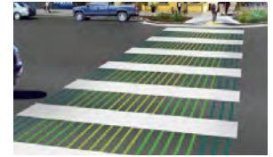
Thermoplastic crossing with custom pattern inlay
