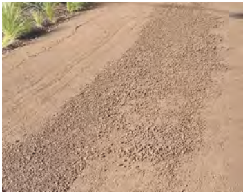
P11: compacted decomposed granite, red-brown pathway mix
