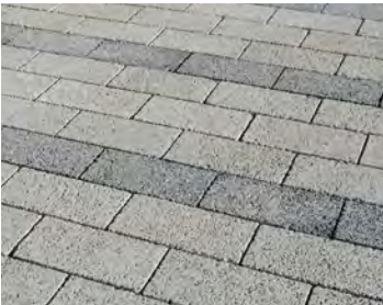
P3: pervious concrete paving with grind finish
