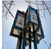
12 reinstall lamp posts
