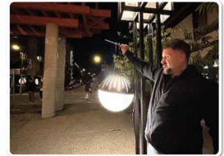
Option 3: 12" Zume, 42" spacing, 14' high -metal shade color options -adjustable color and temperature
