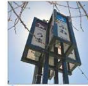
12 reinstall (5) lamp posts
