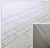
4 stone paving w/ metal inlay accents
