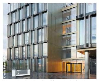
The use of vertical shifts add visual interest by breaking the façade into smaller vertical elements. These shifts should relate to the location and proportion of interior programmatic uses.
