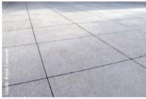
Enhanced Cast-in-Place Concrete with Saw-Cut Joints
