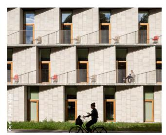
Sawtooth balconies or bay windows reduce the visual mass of the streetwall by introducing a pattern of smaller-scaled components. They can be open, partially enclosed, enclosed, projections, or recesses from the main façade.
