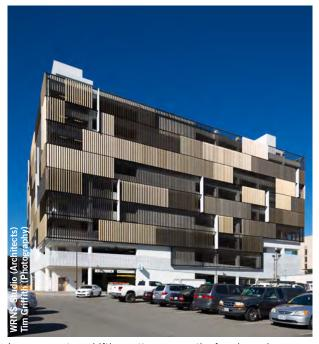
Louvers create a shifting pattern across the façade, and modulate scale. They also redirect light from the headlights of cars to create a dynamic building when in use.
