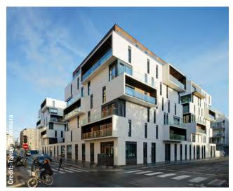
Projections help create shadow lines and added façade depth. Such projections should be located and scaled to relate to interior programmatic uses.
