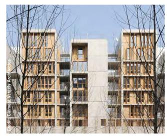
Volumetric notches add visual interest by introducing vertical recesses into the massing of the streetwall. The notches should correspond to the delineations between individual units, balconies, or porches.
