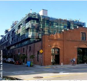
The addition above the existing building uses a vertical hyphen in conjunction with balconies and recesses.
