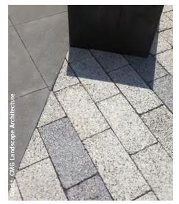
PERMEABLE CONCRETE UNIT PAVERS
