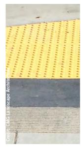
DETECTABLE SURFACE PAVING - SF Public Works STANDARD
