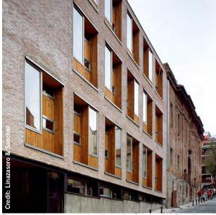
Recesses help create shadow lines, depth, a sense of quality, and durability.
