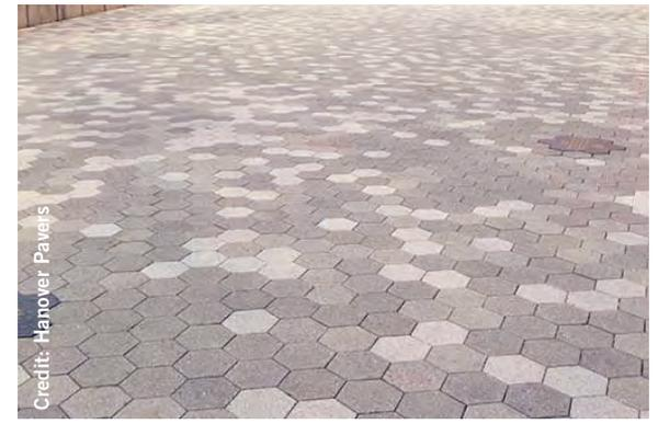
Pre-cast concrete unit pavers and pre-cast permeable concrete unit pavers.
