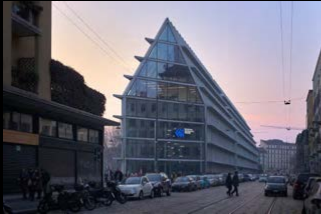
327_Feltrinelli, Milan - Concrete Frame
