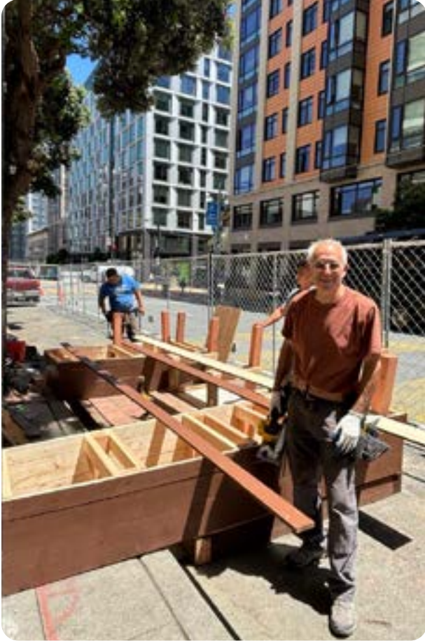
Jeff Miller and company commencing parklet construction in front of 111 Jones.
