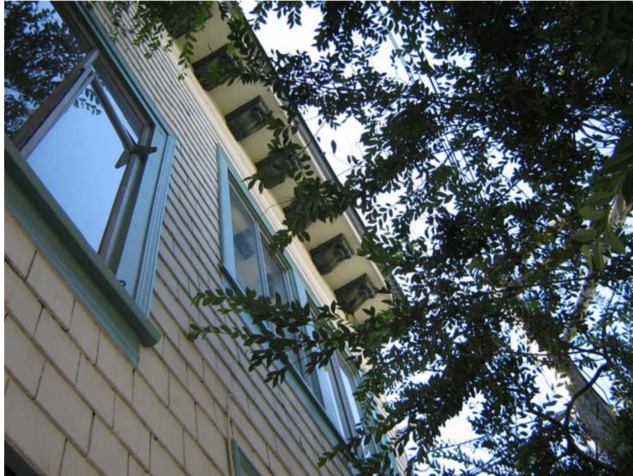
Detail, upper story and roofline
