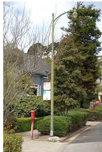
Example of streetlight on Montalvo Avenue. (Note the teardrop globe has often been retrofitted with a cobra light.)
