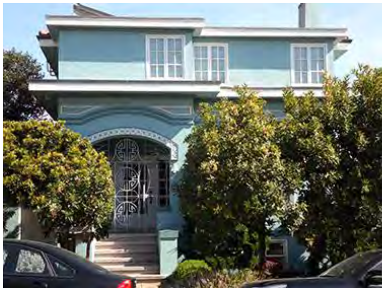
414 38 th Avenue. Designed by Ida McCain for builder S. A. Born.
