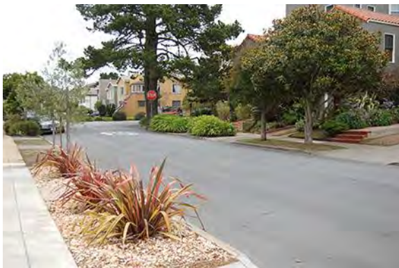
Example of typical sidewalk and planting strips.
