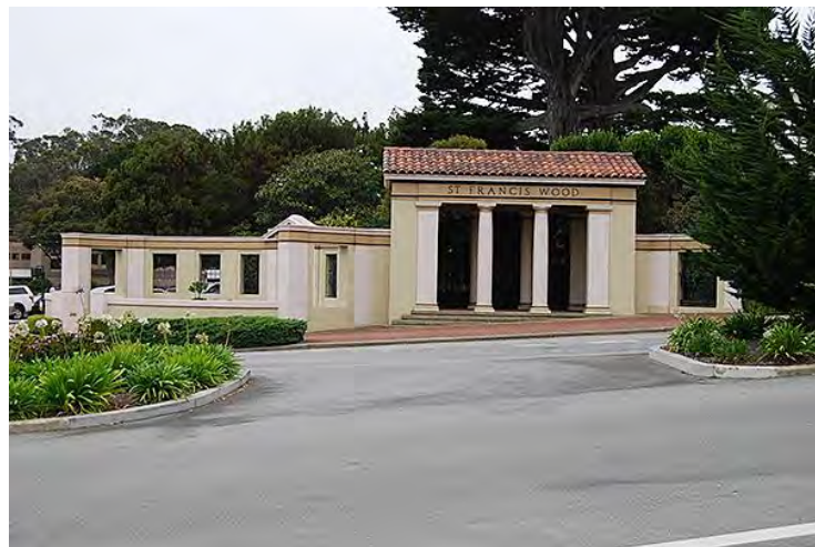
North side of Main Entrance at St. Francis Wood and Junipero Serra Boulevards.
