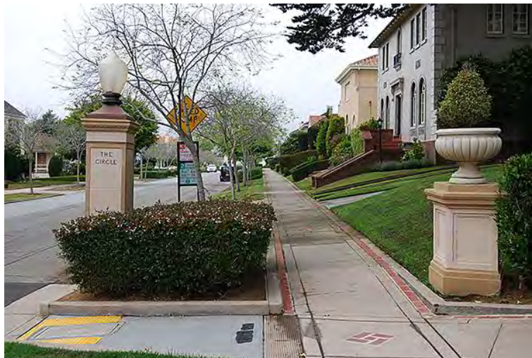
Set of pillars that frame sidewalks at the intersection of St. Francis Wood Boulevard and Santa Ana Avenue.
