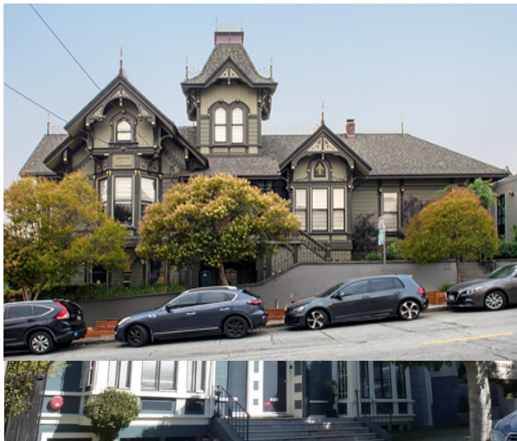
Fig. 17. 1020 Pierce Street in San Francisco (ca. 1885) displays characteristics including decorative bargeboard and lancet windows. (Source: Google Maps, 2023)
