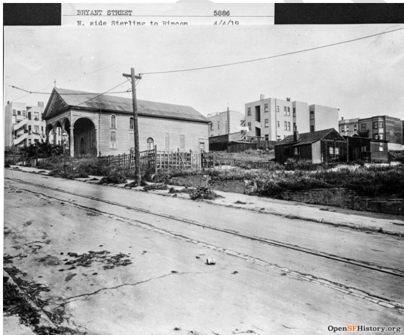
Fig. 7. 1919 photo of St. John Prodromos Greek Orthodox Church and Alexander the Great Meeting Hall (non-extant), 37 Sterling (near now Bryant Street onramp to the Bay Bridge). Property displays Greek Revival features including the full-width porch with columns. (Source: OpenSFHistory / wnp36.02100)
