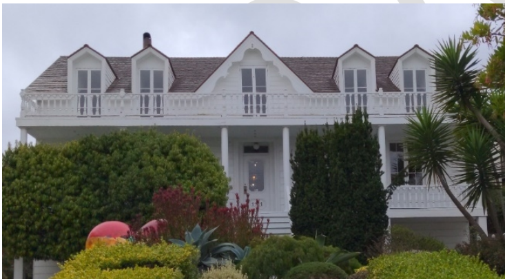
Fig. 16. Abner Phelps House, 1111 Oak Street (Landmark No. 32), constructed ca. 1850 is one of San Francisco's earliest examples of the Gothic Revival style. Note carved bargeboard and steeply pitched roof. (Source: San Francisco Planning Department, 2024)
