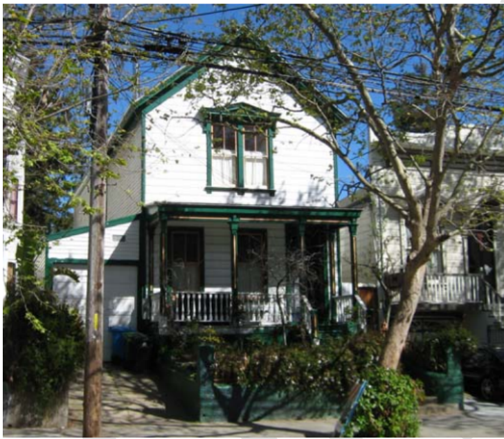
Fig. 9. 727 Shotwell Street , ca. 1868. Greek Revival elements include the columned full width front porch, and bracketed pediment above the second story windows. (Source: Page and Turnbull, 2008)
