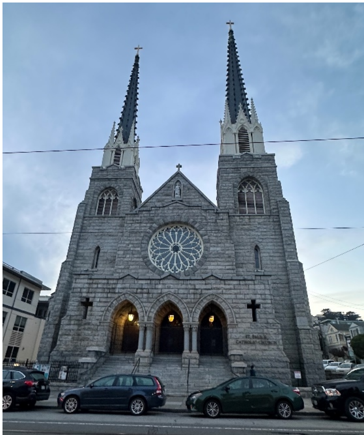
Fig. 19. St. Paul's Church at 1660 Church St. includes stone cladding, lancet openings, two towers with spires, and more. The structure was constructed in 1901 as the style continued to be popular for religious structures in the 20 th century. (Source: San Francisco Planning Department, 2024)
