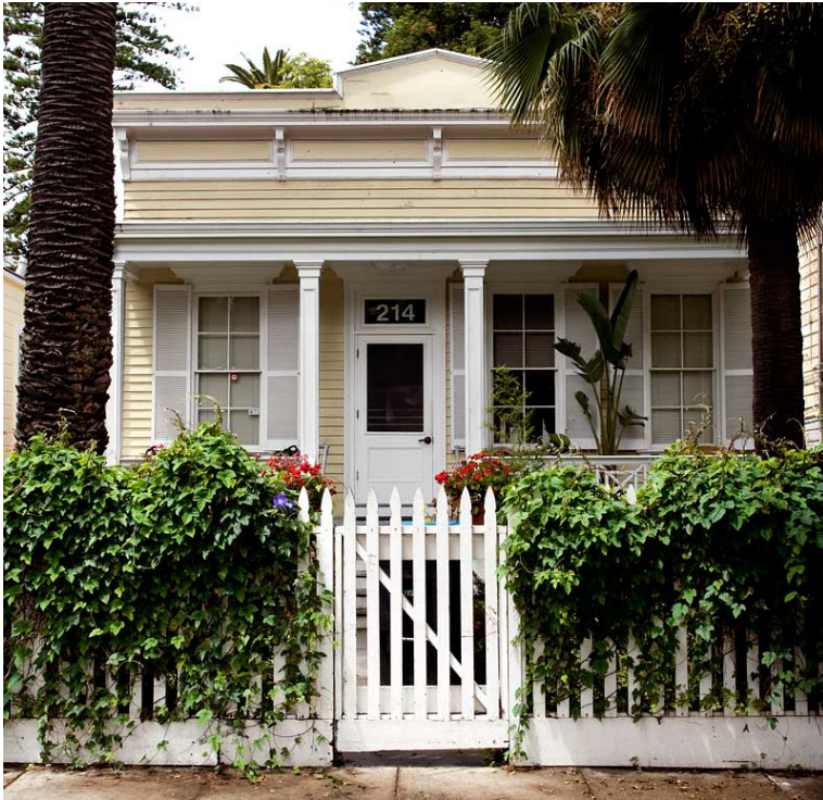
Fig. 8. Tanforan Cottage, 214 Dolores Street (right), ca. 1854, Landmark No. 67. Located near the Mission District this residential property, along with the neighboring Tanforan Cottage at 220 Dolores Street, Landmark No. 68, built around the same time, showcase elements of the Greek Revival style with the prominent, flattened window crowns and substantial window frames. The classical porch appears to have been modified. (Source: Google Maps, 2015)
