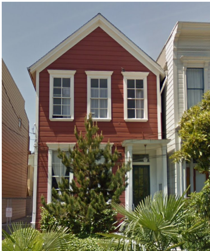
Fig. 10. 858 Shotwell Street , ca. 1866. Greek Revival elements include the square columned front porch, gabled roof and wood windows with divided lites and flattened surrounds. (Source: Google Earth, 2011)
