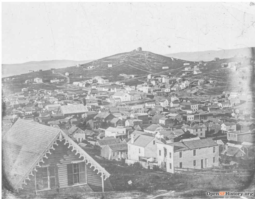
Fig. 12. View from Russian Hill, circa 1860. Home in lower left foreground displays bargeboard characteristic of the Carpenter Gothic style. (Source: OpenSFhistory wnp13.199)
