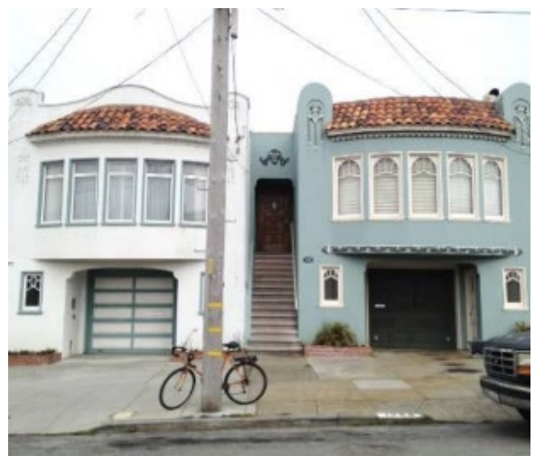
Figure 19. 1434 and 1438 48th Avenue
