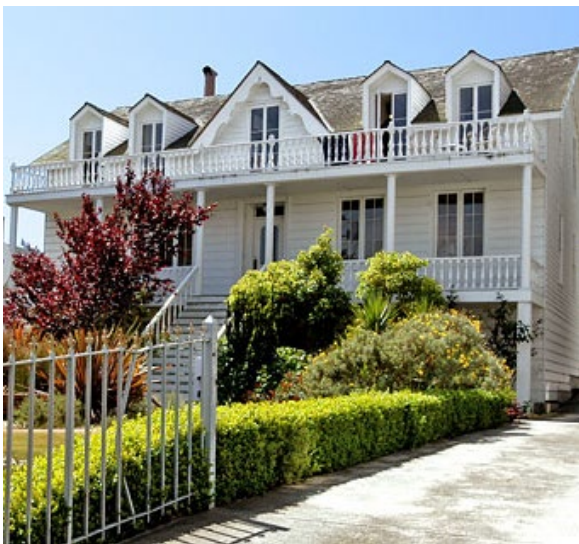
Figure 3. Abner Phelps House, 1111 Oak Street (Landmark #32)
