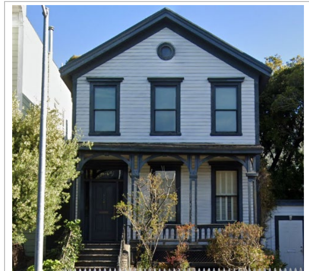
Figure 6. Stanyan House, 2006 Bush St. (Landmark #66)
