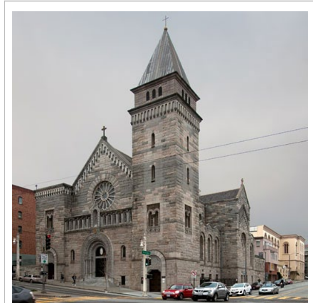
Figure 13. Saint Brigid Church, 2151 Van Ness Avenue (Landmark #252)
