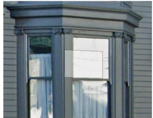
Example of projecting bay window, wood siding, and ornament at windows.
