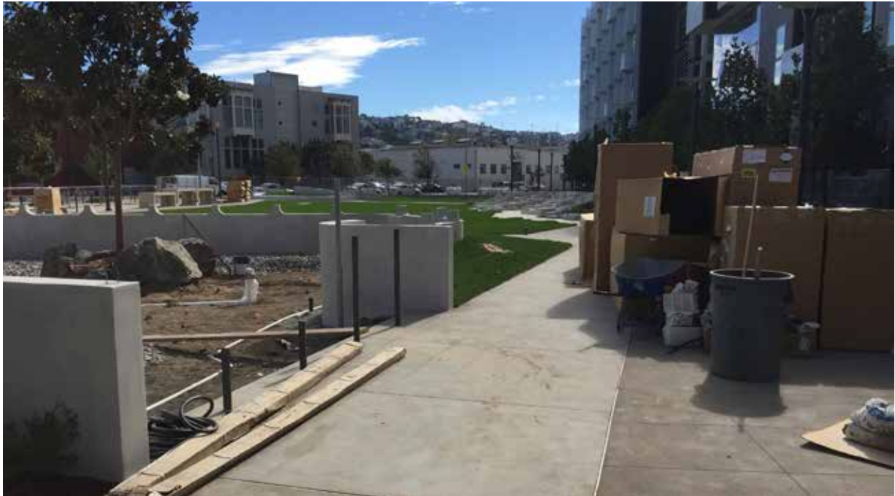
FIGURE 5.2.1 Daggett Park Under Construction
