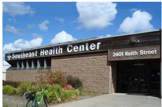
The Southeast Health Center.
