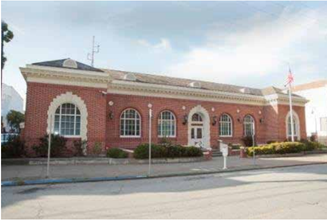
Richmond Branch Police Station. Photo courtesy San Francisco Police Department
