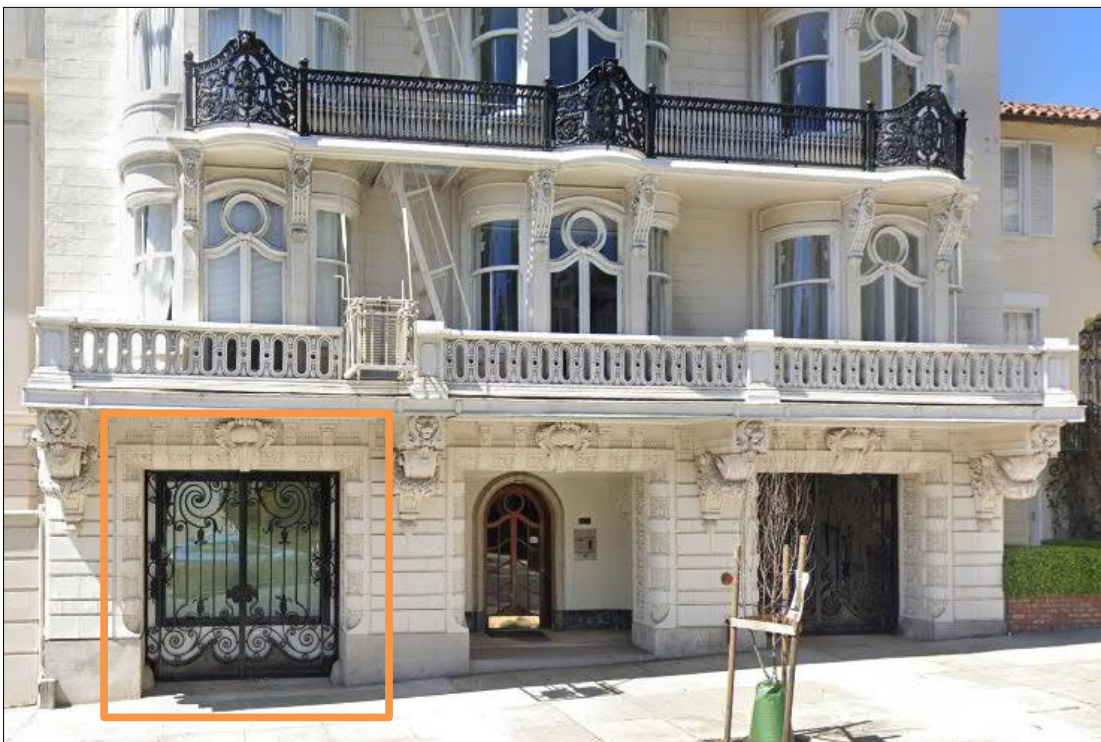
Character-defining elements (gate and surrounding decorative elements) were retained. Garage gate was re-purposed for residential use via insertion of glazing.
