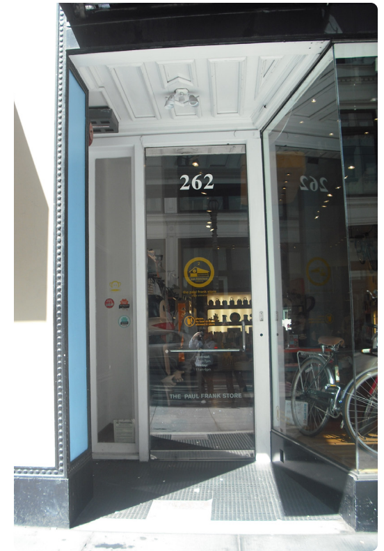
Historic paneled vestibule ceiling at the storefront entrance
