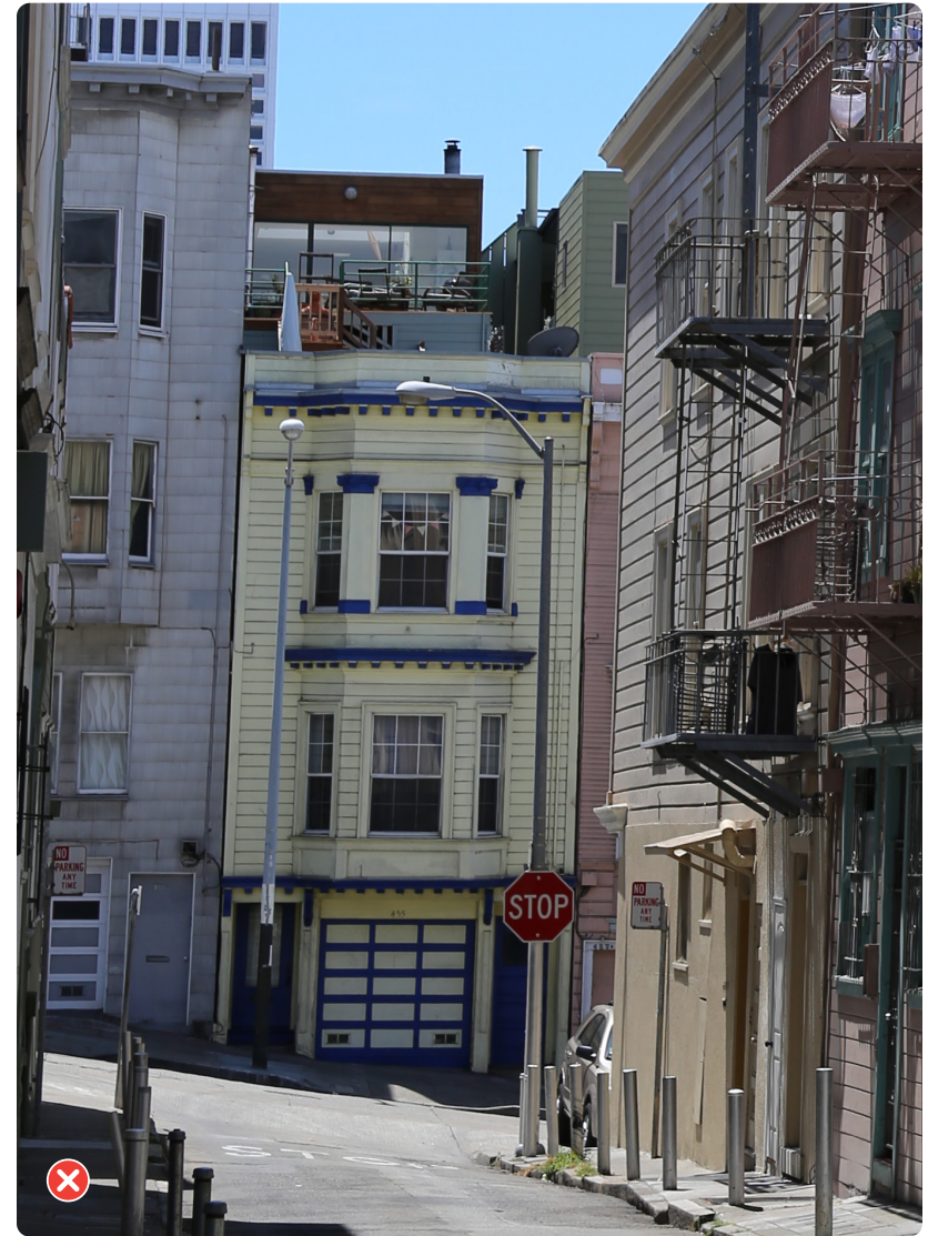
The windows of this visible addition to a historic building do not align with the placement or vertical orientation of the historic building, and the addition's solid-to-void ratio is not within 10 percent of the original building's solid-to-void ratio.
