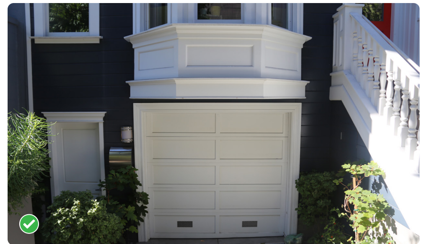
A garage insertion that did not require modification of the historic bay window and is recessed from the surrounding wall surface
