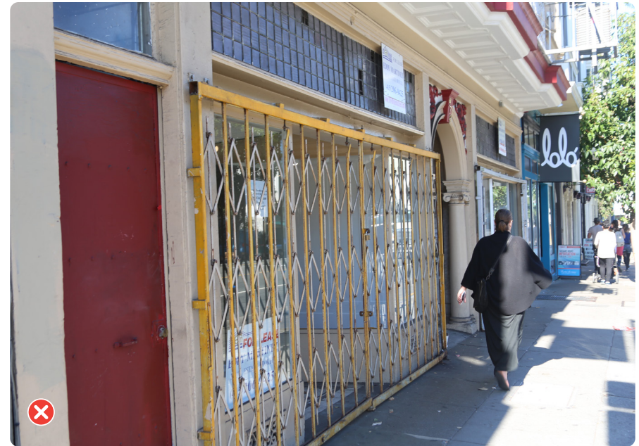
This security gate is mounted on top of a historic storefront with a highly visible frame rather than being installed within the storefront opening.
