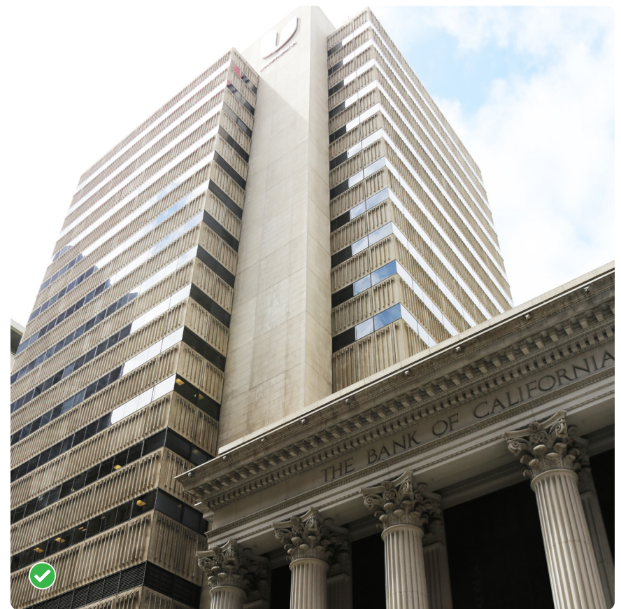
The concrete cladding of a 1968 tower addition to 400 California Street matches the texture and finish of the original 1908 building's granite façade.
