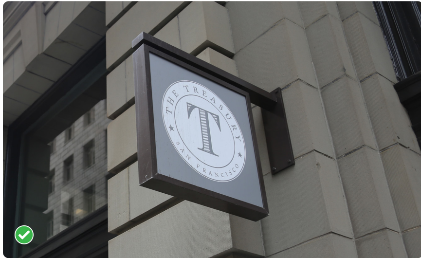
Projecting sign appropriately installed in the mortar joints
