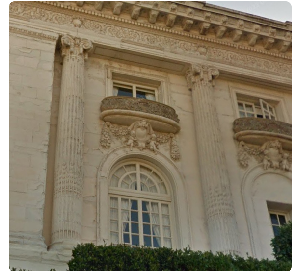
Historic windows at 2080 Washington Street
