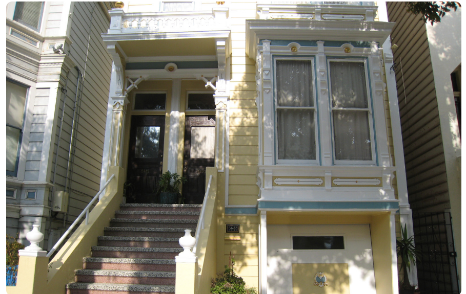
Historic moldings, ornamentation, recessed garage doors and bay window retained.
