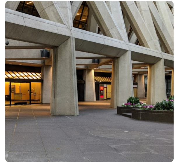
Structural elements at 600 Montgomery Street
