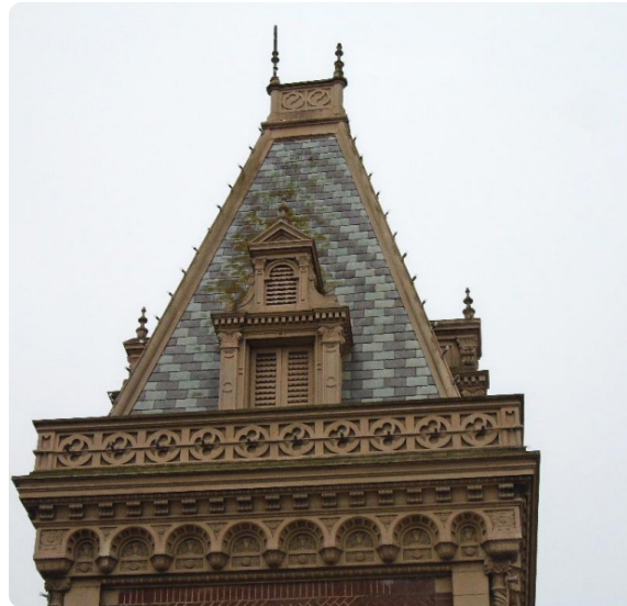
Historic slate roofing material at Ghirardelli Square
