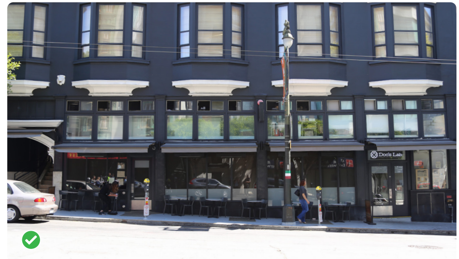
These open-sided, sloped cloth awnings with unframed valances meet the awning standards.
