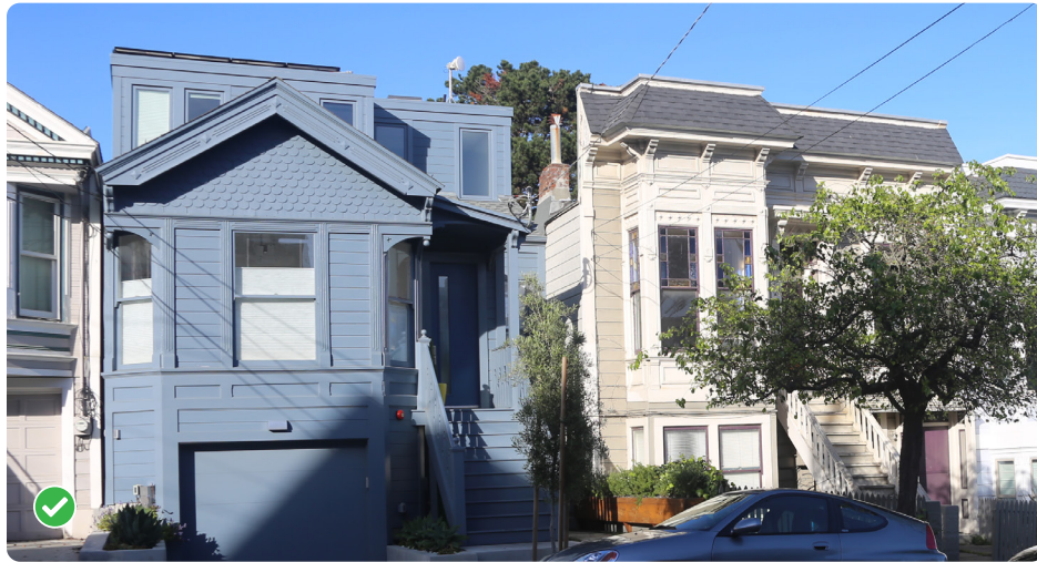
The windows of this historic home's rooftop addition are vertically oriented to align with the vertically oriented windows of the historic home.
