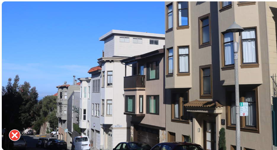
The rooftop addition to the building at the center of this image features a windowless street-facing façade, and the horizontally oriented visible side windows do not align with the vertically oriented windows of the historic building.
