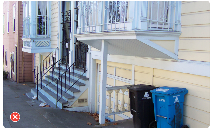
An inappropriate garage insertion that required modification of the historic bay window
