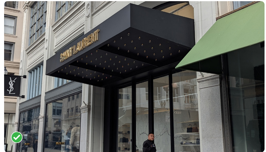
This non-historic marquee meets the preservation standards.
